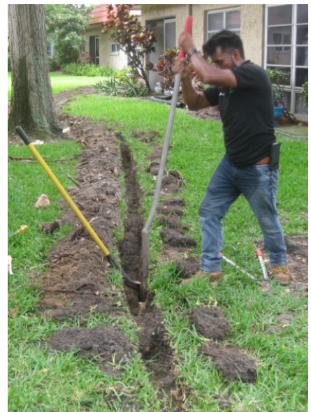
Juan—digging Building 16 drainage
