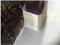
The cracks were filled with a polymer and the posts were caulked where they met the surface of the walkway, then allowed to dry thoroughly. Finally, after several days of prep work, the walkway was painted with a special paint designed for walkways. The results are dramatic. They will do another one soon. Thank you volunteers for a job well done.
